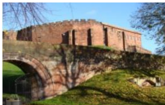
The Chester Walls
